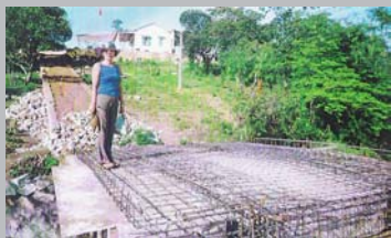
July 2002 Construction of the access bridge
